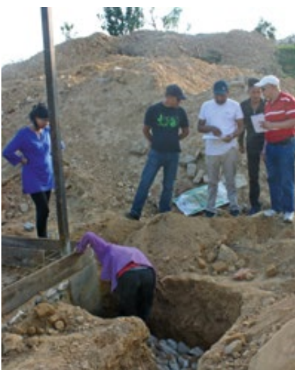
Preparing the construction site
